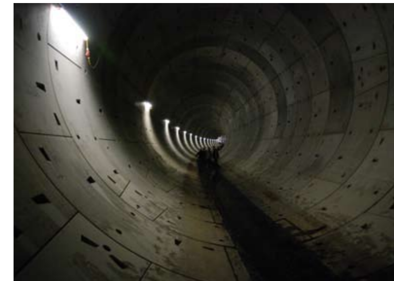
Metro of Leipzig during construction
